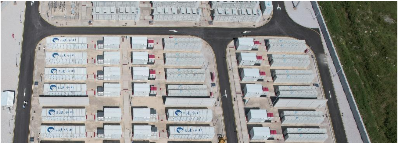
103MW/206MWh Sanxia Water Resources Pingguo Shared Energy Storage Power Station, Guangxi
