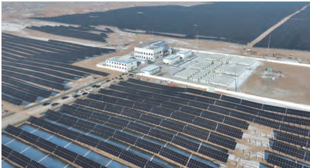
60MW/120MWh Energy Storage Matching for the 400,000-kilowatt Wind-Solar-Storage Integration Base Project of CNNC in Xianghuang Banner
