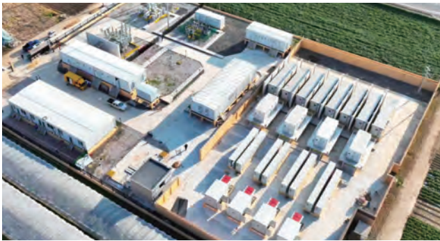
12MW/24MWh Guoneng Electric Power Gaomi Jiaohu Ecological Development Zone Agricultural-Solar Complementary Project with Energy Storage Configuration
