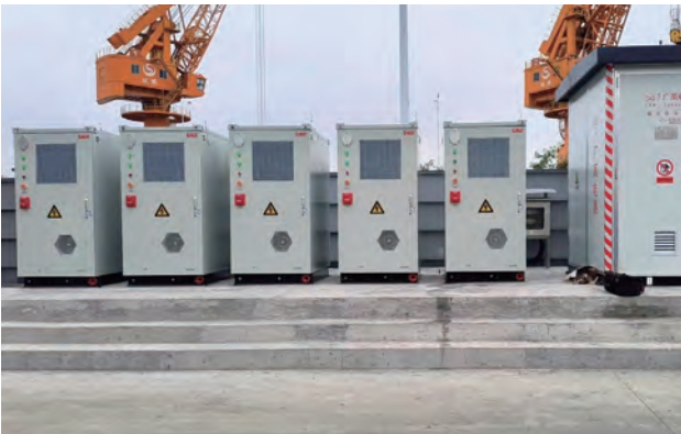
675kW/1305kWh Green Power Renovation Project of the Terminal of Shuangqiao (Guangzhou) Co., Ltd.
