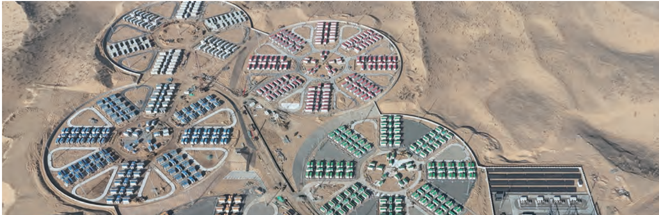
350MW/1400MWh Xinjiang Huadian Urumqi Photovoltaic Base 1000MW/4000MWh Independent Energy Storage
